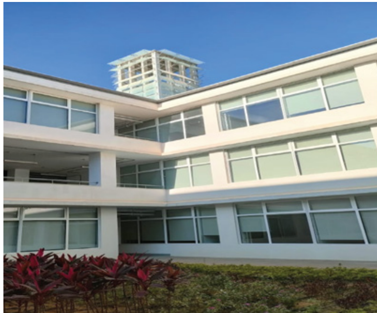
EJUST ventilation system
