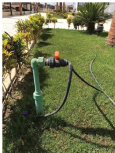
Drip irrigation system to minimize water loss
